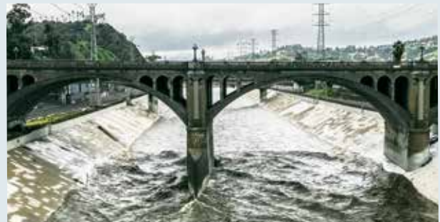
While not a source of Metropolitan supply, the Los Angeles River can generate significant stormwater runoff during wet winters.
